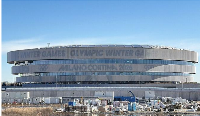
Exterior of Palalitalia (Milano Santa Giulia Ice Hockey Arena), a 16,000-seat arena in Milan - Photograph of Quintin Soloviev, licensed under Creative Commons-Attribution 4.0, via Wikimedia Commons.
